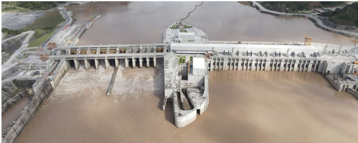
Xayaburi Hydroelectric Power Project
