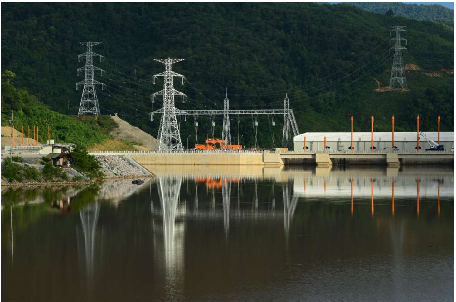
500 kV Takeoff yard and Transmission towers
