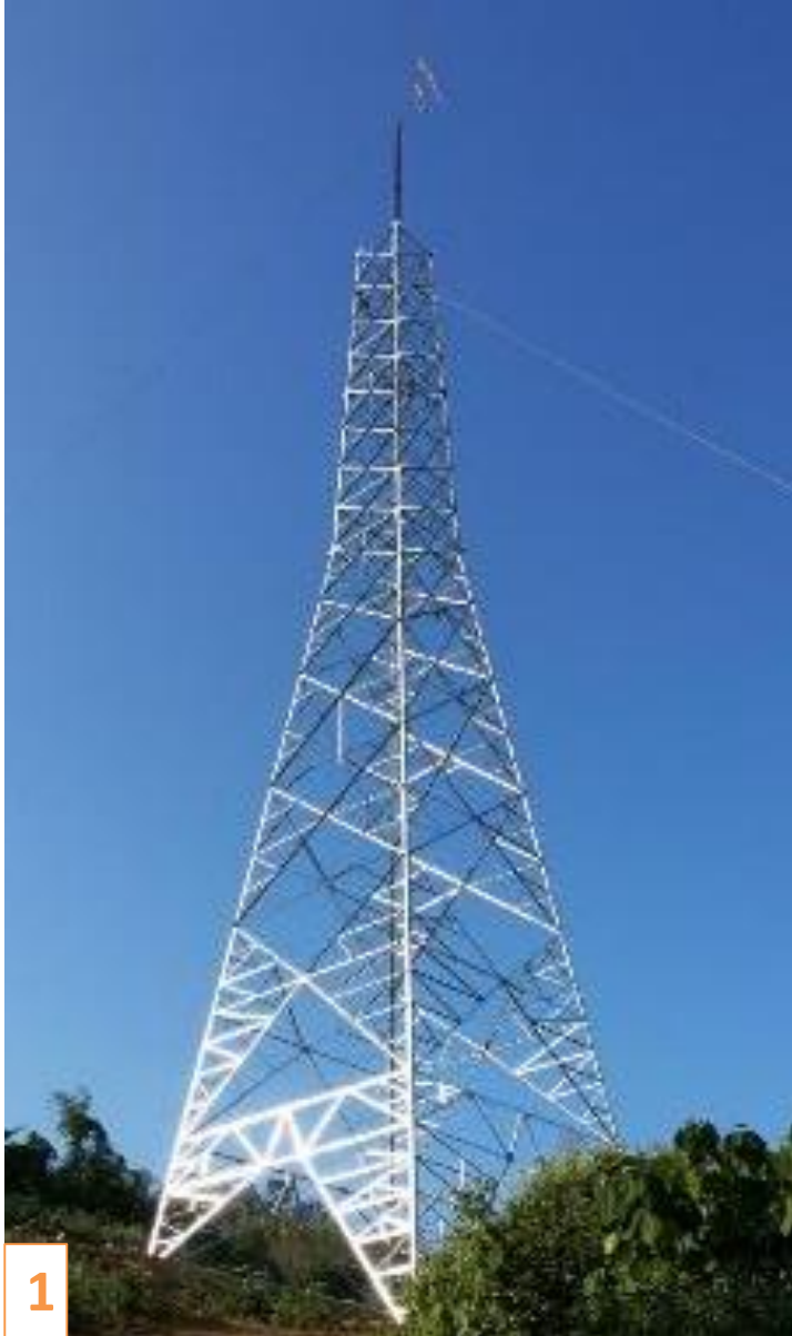
Tower erection (T32A/21)
