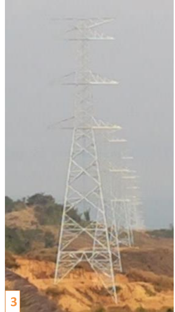
Completed tower erection Section 2
