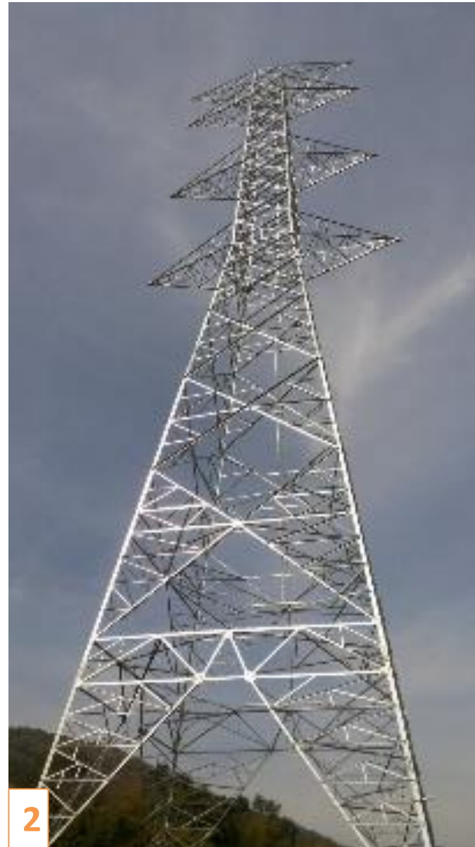
Tower erection (T31/9)
